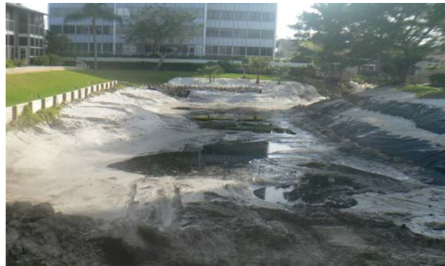
Pond 2 – Construction Phase
