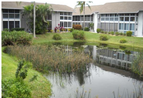
Pond 1 – Existing Conditions
