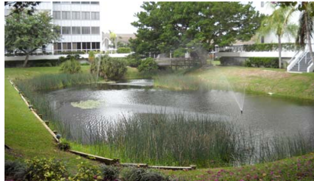
Pond 2 – Existing Conditions
