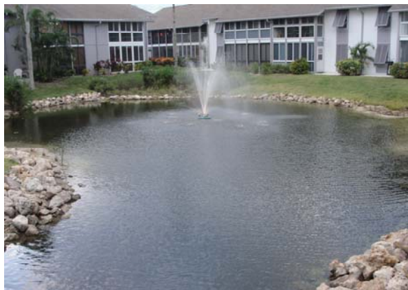
Pond 1 – Post Construction
